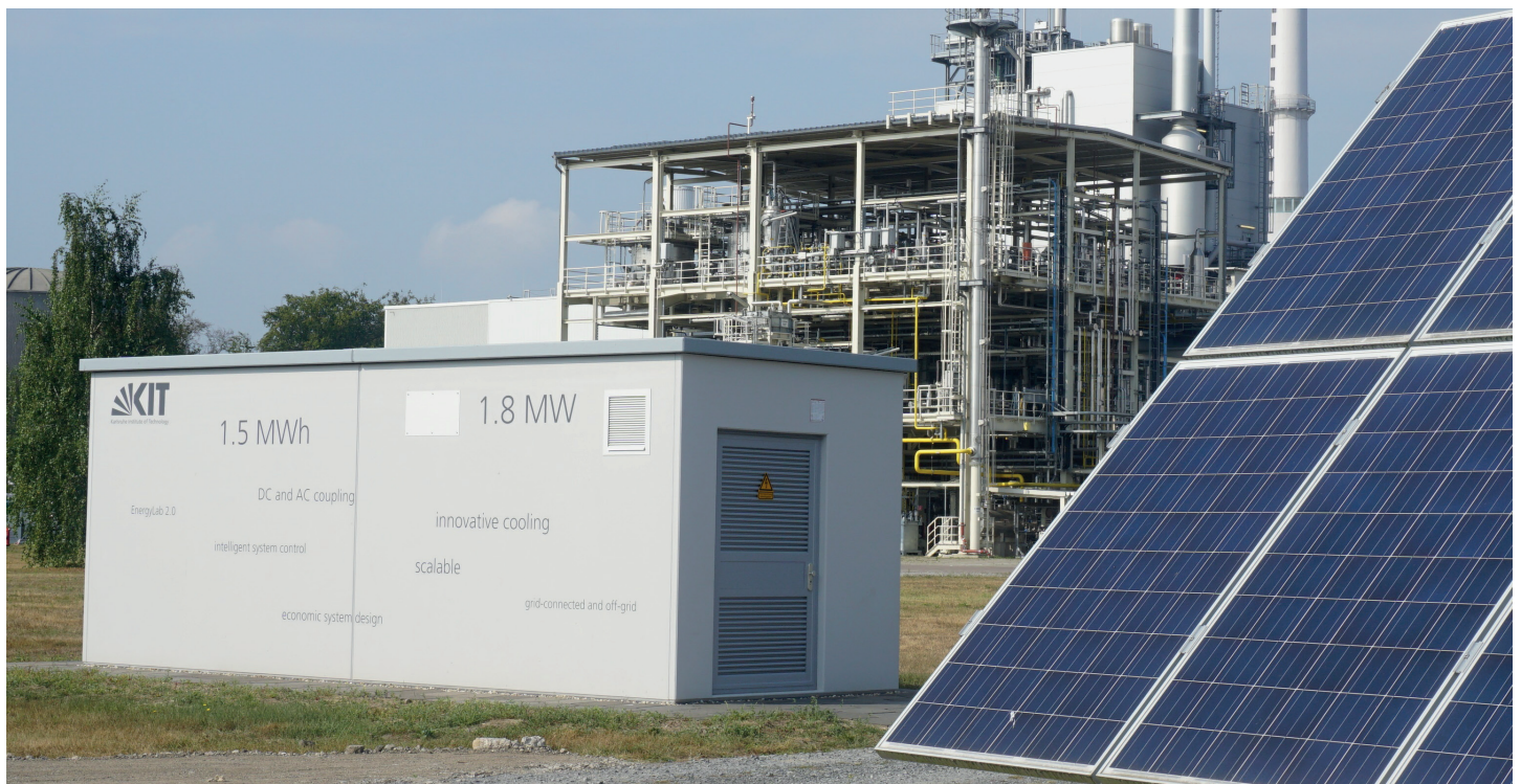
Large-scale storage at the KIT PV storage park
