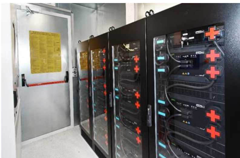
The batteries store solar power and feed it into the mains of HIU, if required. (Photo: Frederik Elschenbroich, ads-tec)
