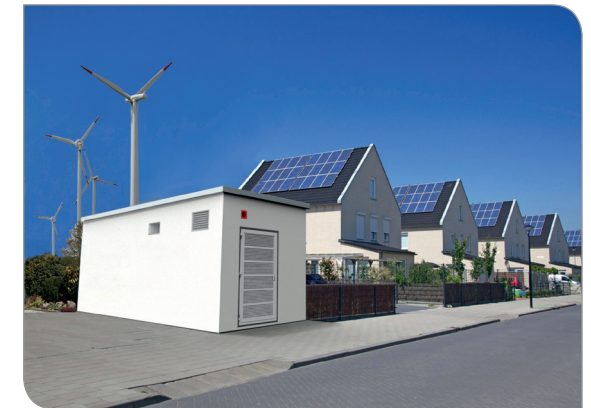
KIT Large-scale energy storage for a residential areas (build_up design)
