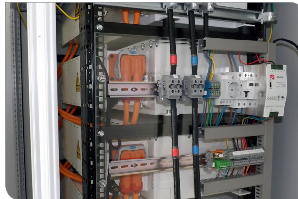
AC-coupled battery storage system at KIT
